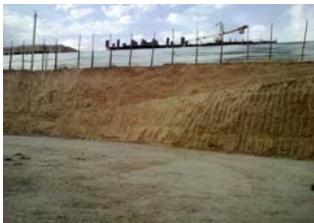
Figure 9 Gravel-sand cushion, made to one level
