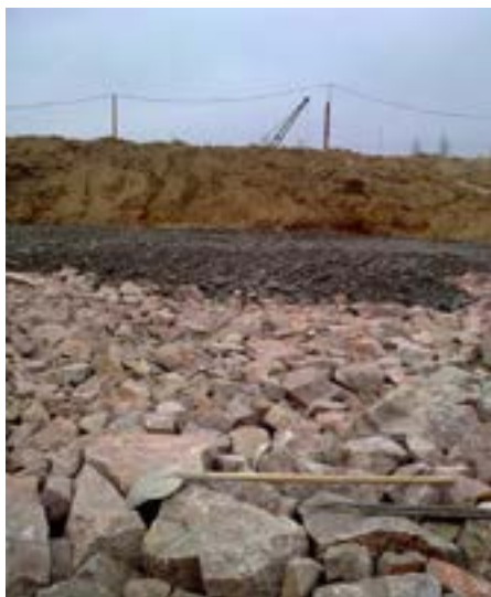
Figure 1. View of a two-layer embankment made of rubble stone and gravel.
